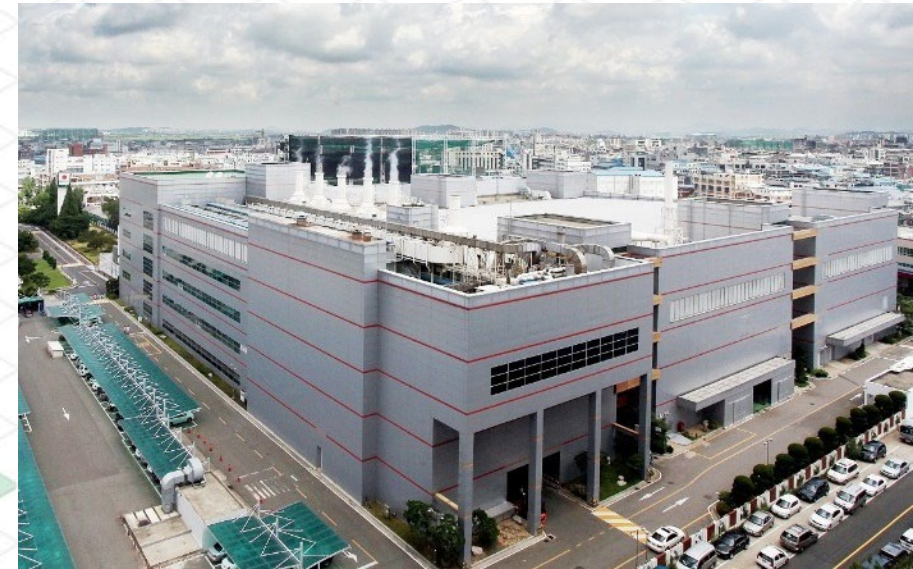
Above: a DB HiTek plant
